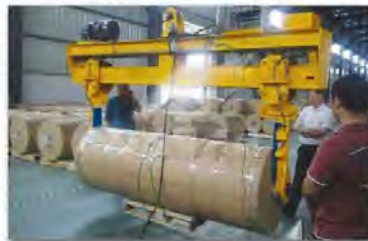
现场安装调试 On-site installation and debugging
